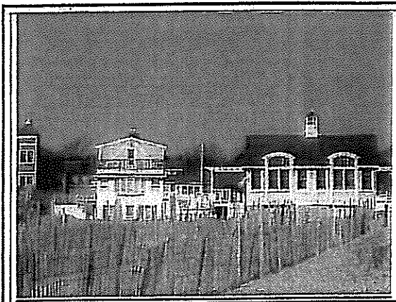
Exterior View of Subject
